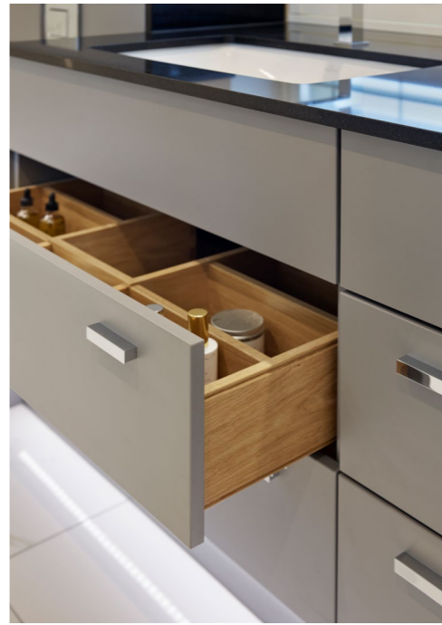
U-shaped drawers wrap around plumbing from sinks and can be sectioned with wooden dividers for organising, utilising the space available to maximum effect.
