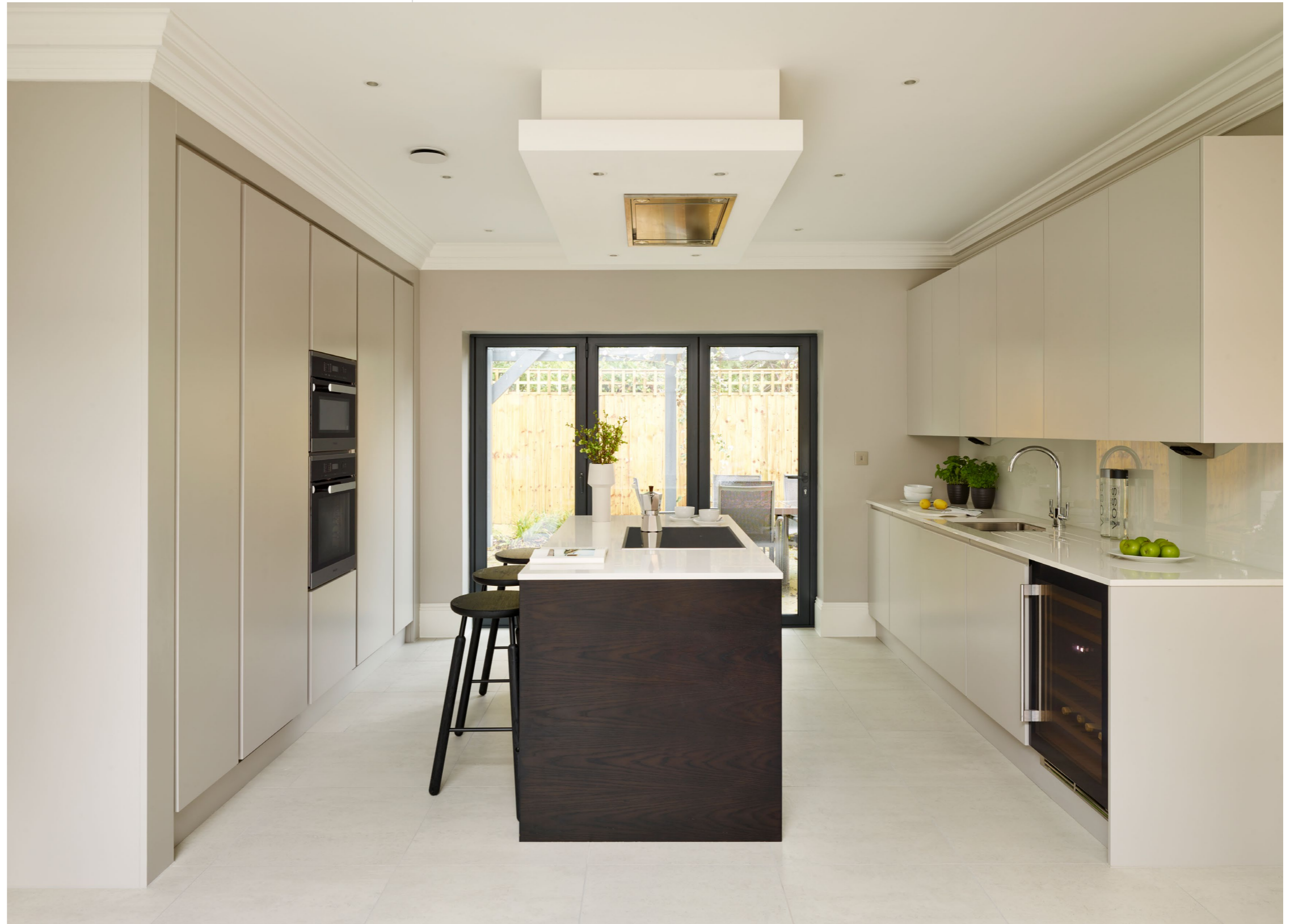
Bulkheads help to house ceiling extractors in rooms where there is not enough space in the ceiling voids, like the one in this kitchen which mirrors the shape of the island.
