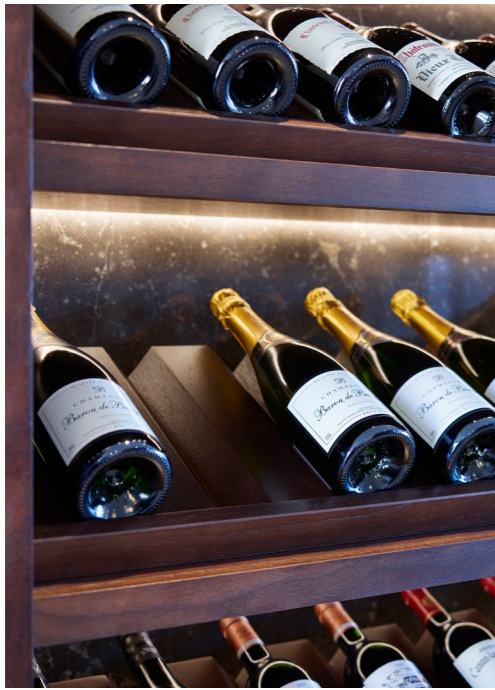
Special angled shelves with v-shaped sections to store bottles can create a beautiful feature when combined with lighting and stone back panels.
